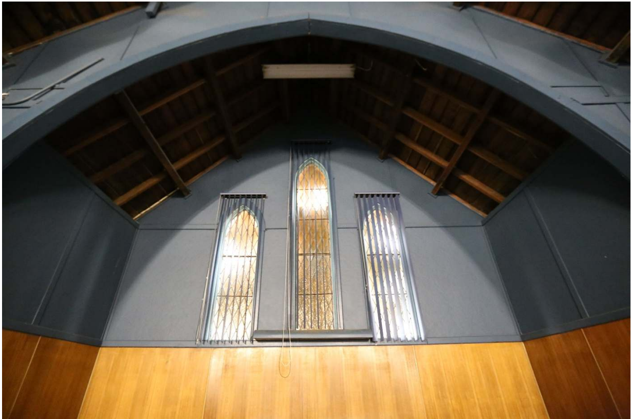
Figure 29. View to apse windows.
