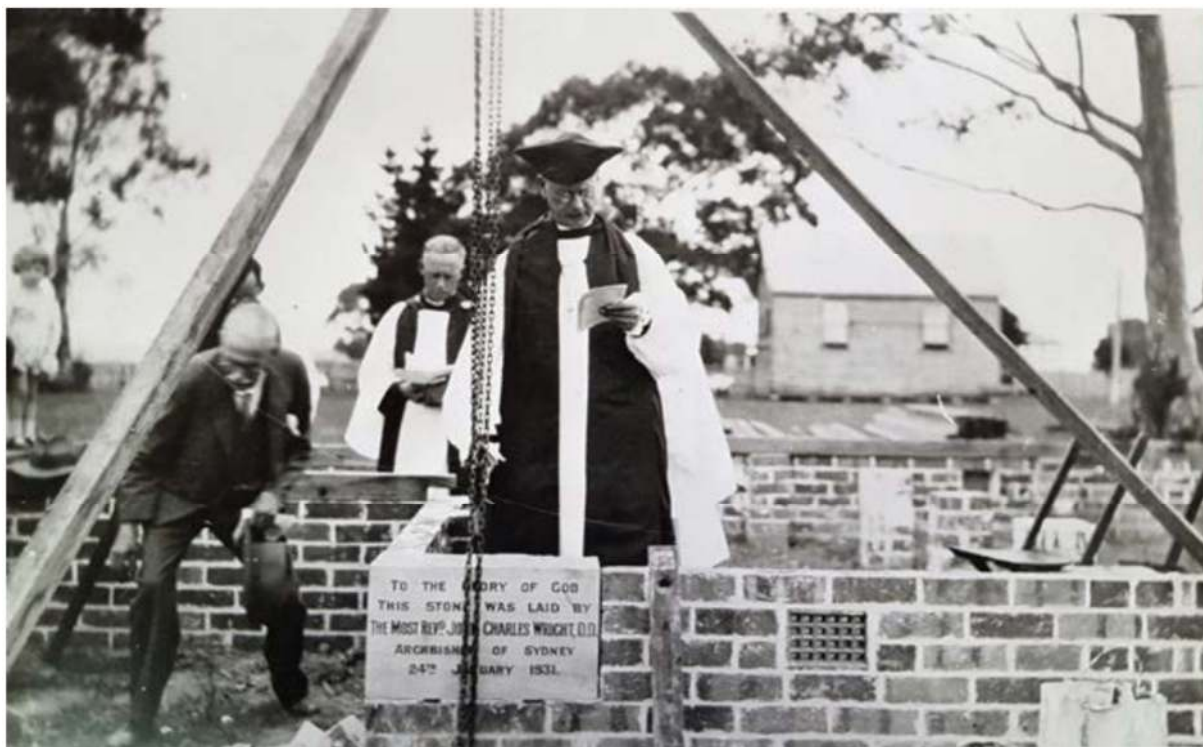
Figure 15. Laying of foundation stone at Holy Trinity Church, 1931. The old church is visible to the right in the background. Source: National Trust.
