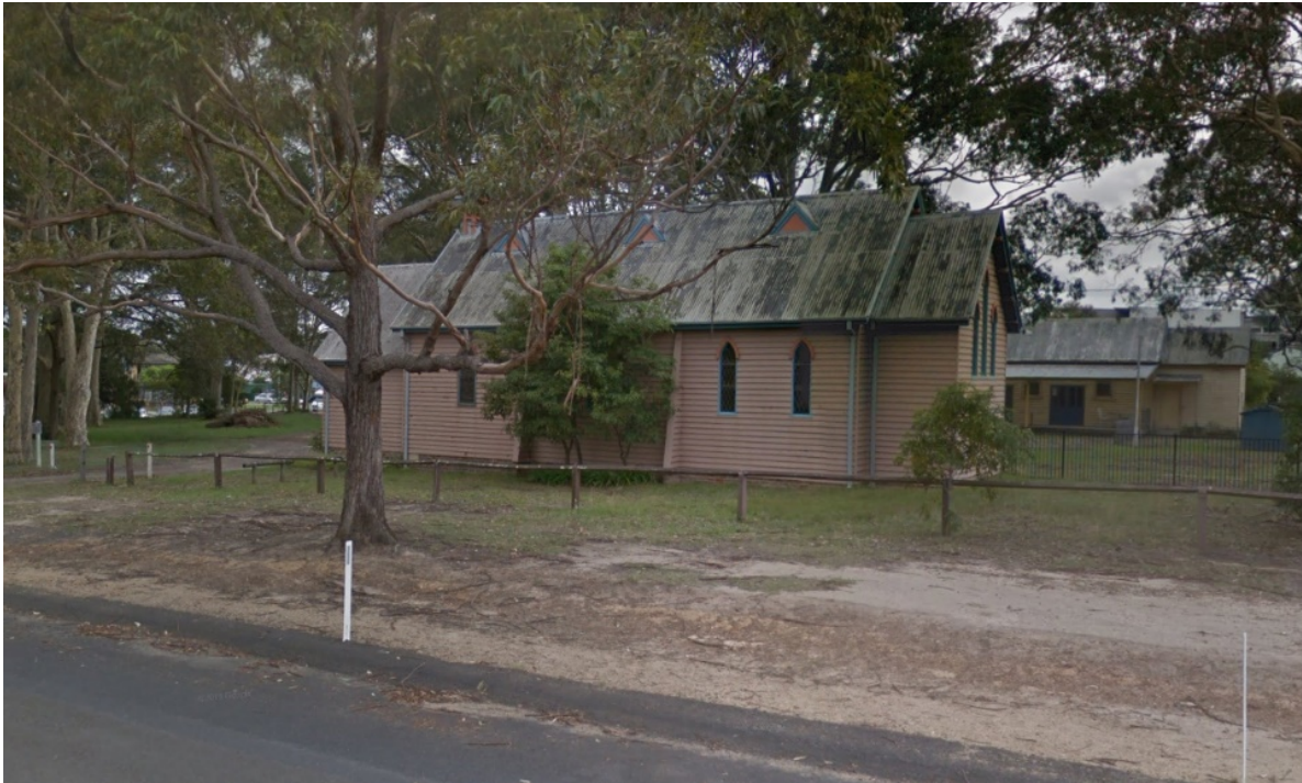
Former Holy Trinity Anglican Church, Huskisson, South Elevation (Source: Google Streetview April 2018)
