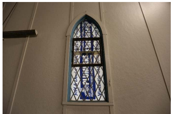
Figure 36. Window on northern wall.
