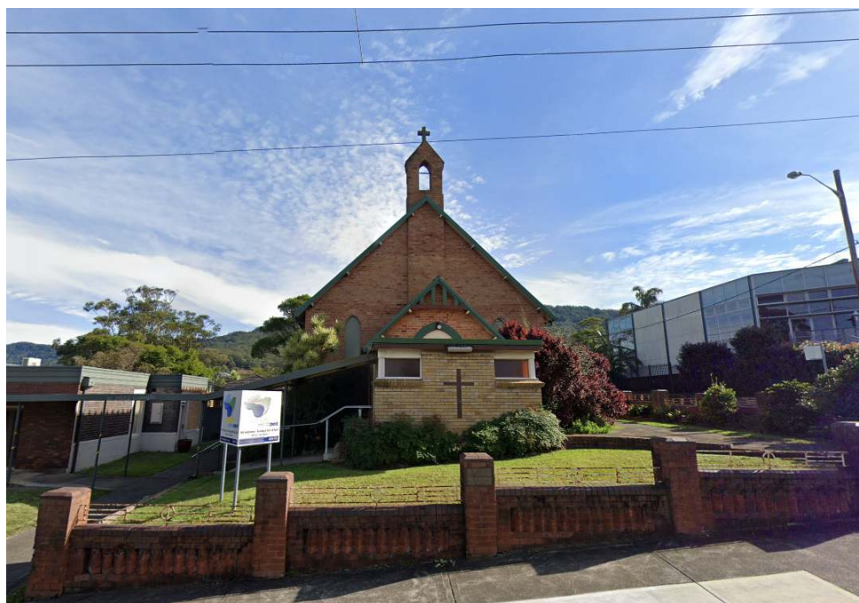
Figure 94. Corrimal Anglican Church. Source: Google Streetview 2021.
