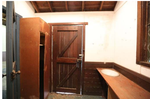
Figure 38. Vestry. Door to church on left, external door in centre.
