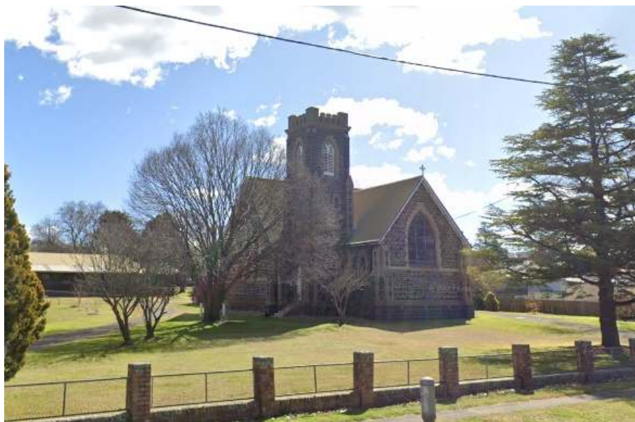
Figure 98. Glen Innes Anglican Church. Source: Google Streetview 2022.
