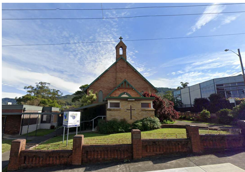
Figure 94. Corrimal Anglican Church. Source: Google Streetview 2021.
