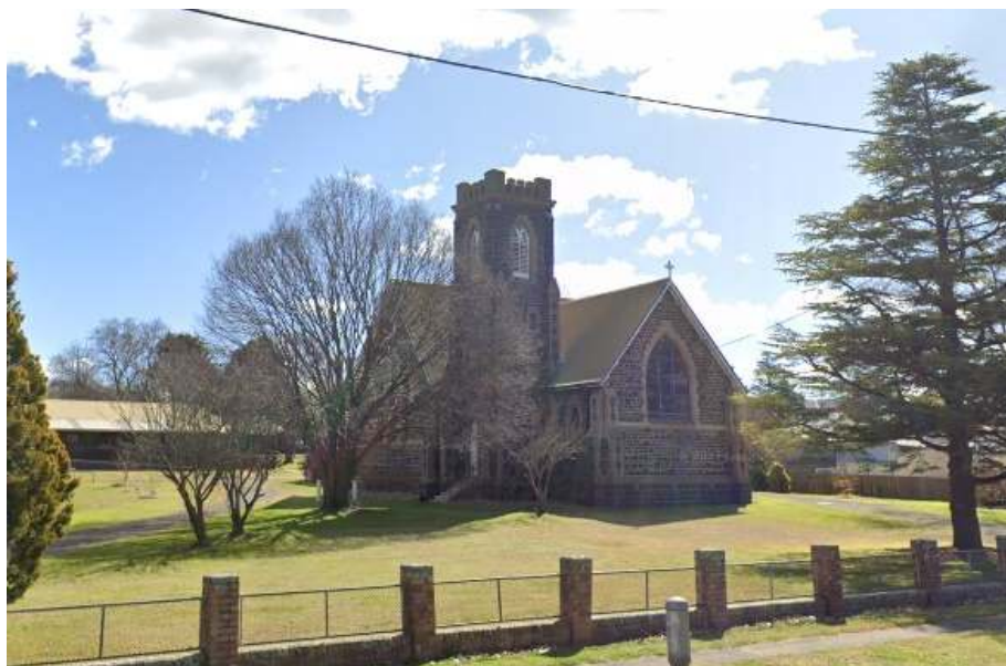
Figure 98. Glen Innes Anglican Church. Source: Google Streetview 2022.
