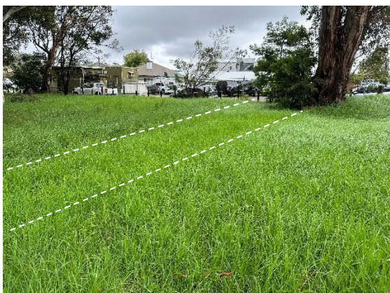
Figure 68. Strip of discoloured grass running north to south (white dashed line), likely associated with drainage (natural or manufactured) in the northern portion of Lot 8, facing north-west.
