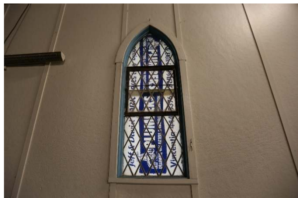
Figure 36. Window on northern wall.
