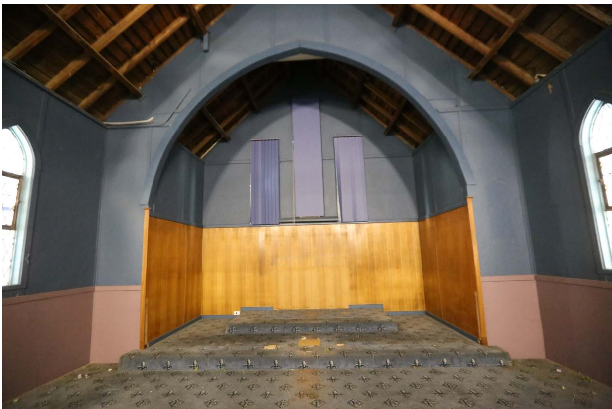
Figure 28. View to apse.
