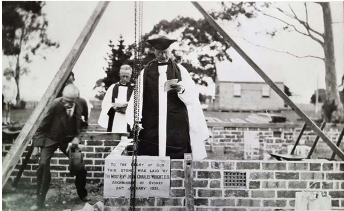
Laying of the foundation stone (1931) Cyril Blacket leaning forward. The original building (now the hall) is in the background. (Source: Heritage Management Strategy)
