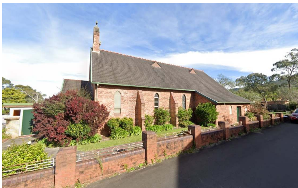
Figure 93. Corrimal Anglican Church. Source: Google Streetview 2021.
