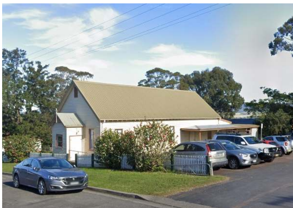
Figure 92. Milton Church Hall. Source: Google Streetview 2021.
